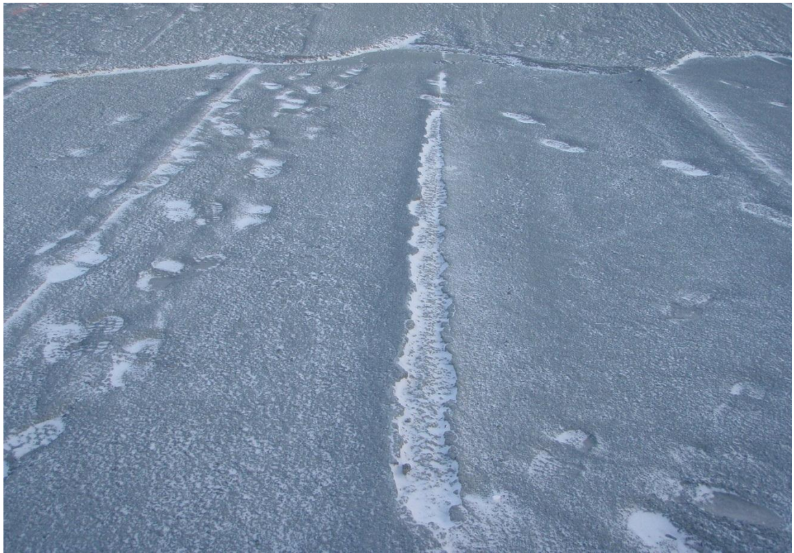
Photo 6: Some hand chipping was completed to eliminate air voids in the previously placed lift.
