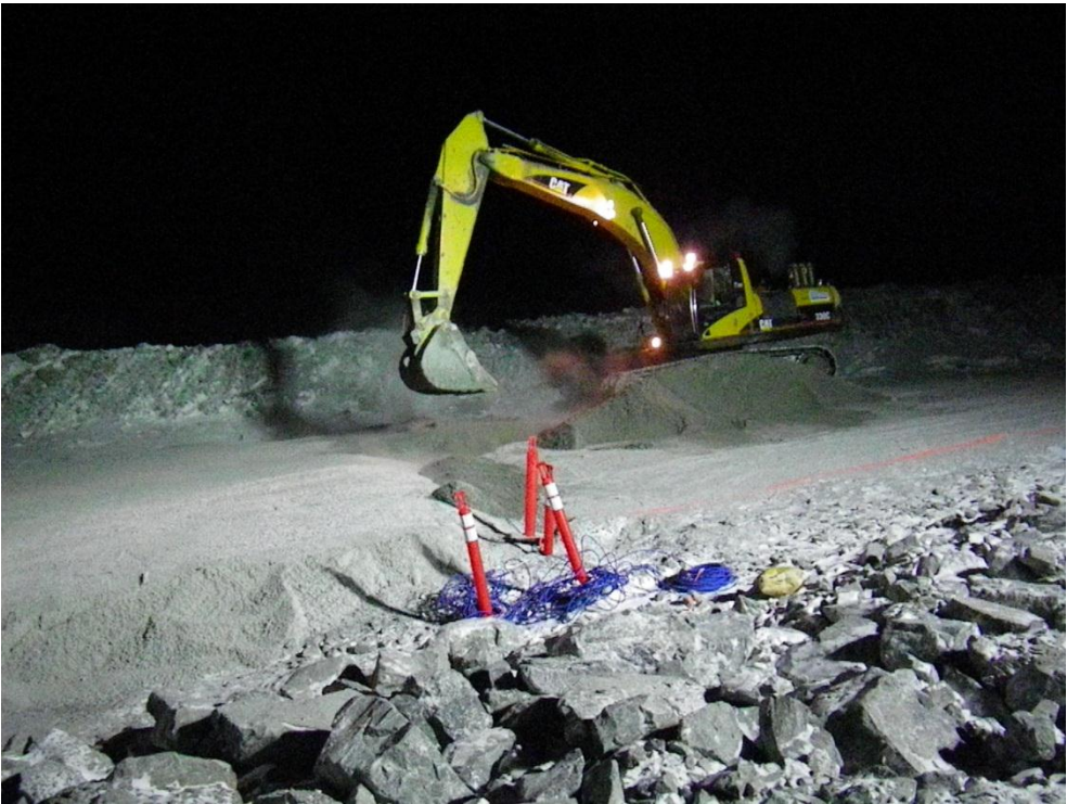
Photo 11: CAT 330 excavator placing FCM over thermistor cable at 0+60.
