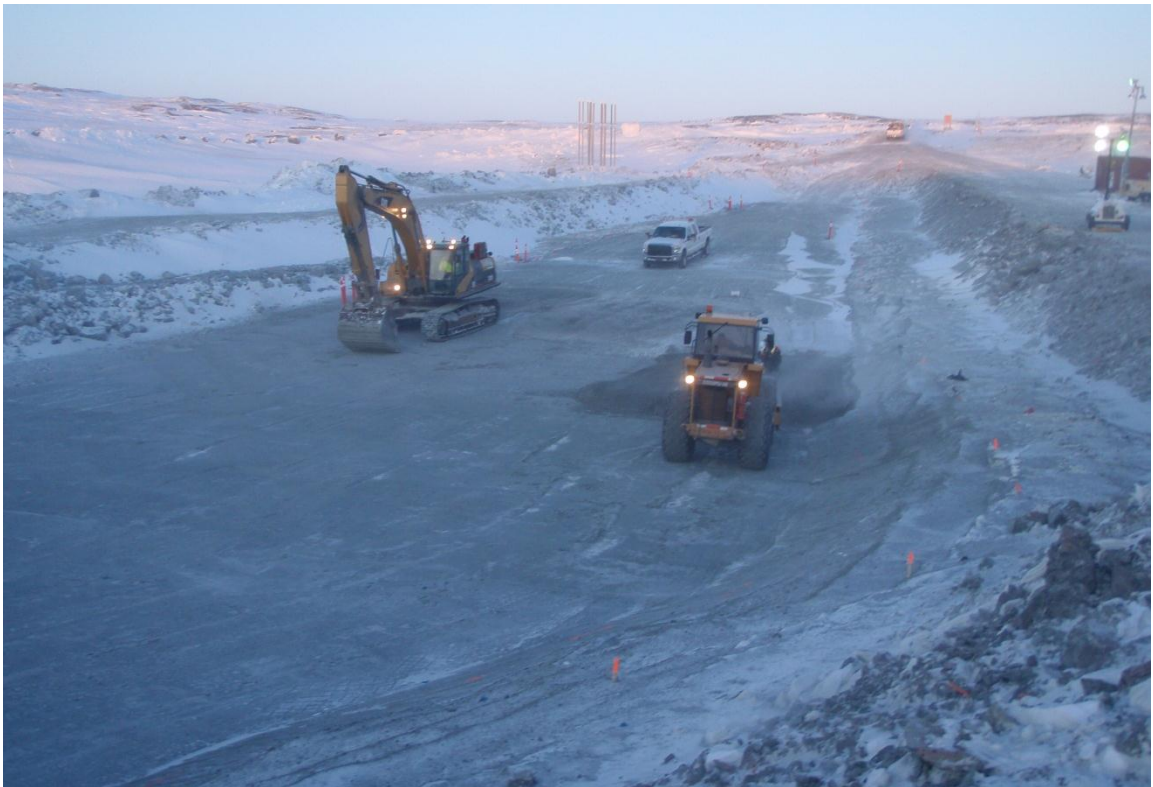
Photo 9: Pickup truck parked immediately before starting placement. Visible freeze back of surface crust was noted within a couple hours of placement.
