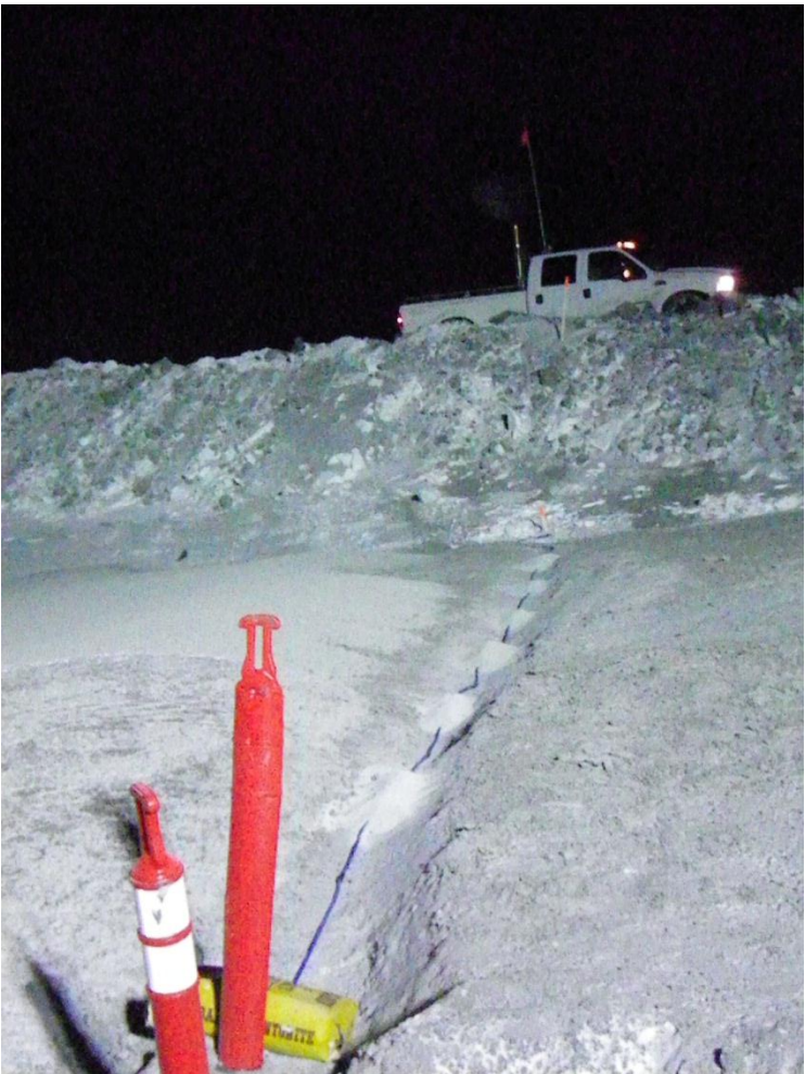
Photo 13: Thermistor cable ND-HTS-060-31.1 laid out with water stops in place ready to be covered with FCM.
