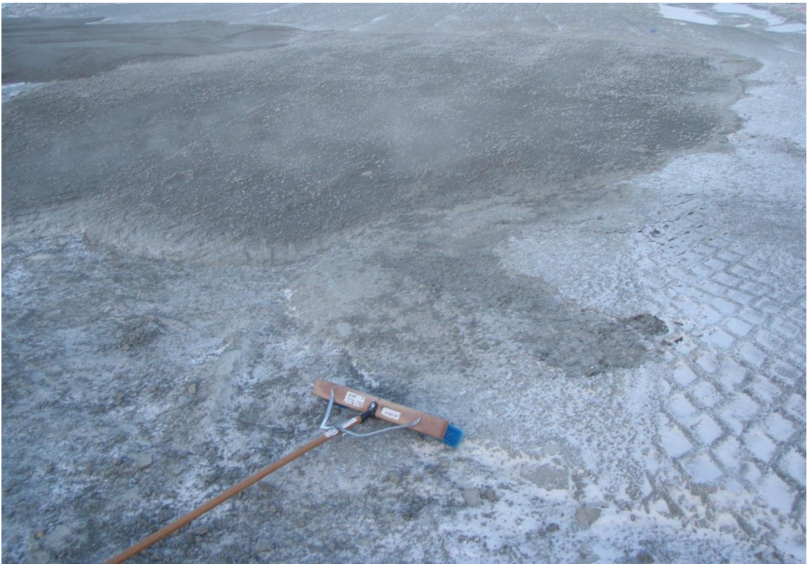
Photo 7: Clean up completed after the packer drove over partially frozen ground. All loose pieces were pull out and the surface was swept before the next tie-in.
